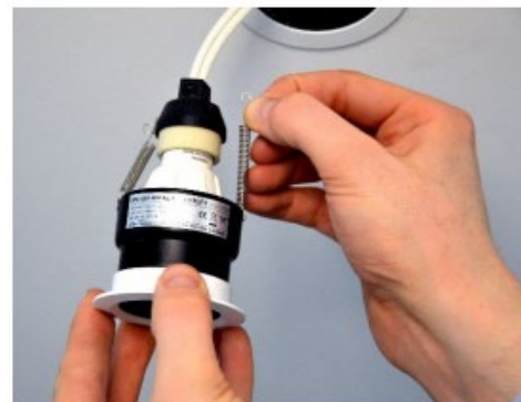
4.6 - Remove the retaining spring on both sides
