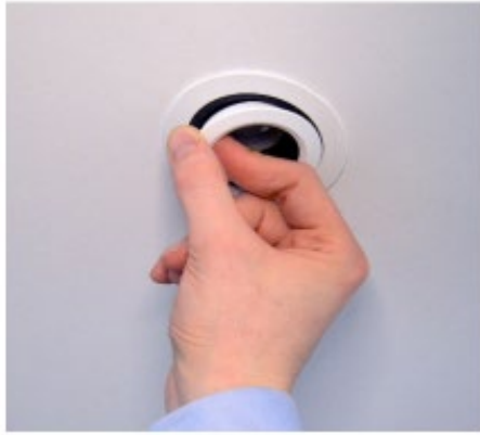
4.3 - separate the magnetic inner fitting
