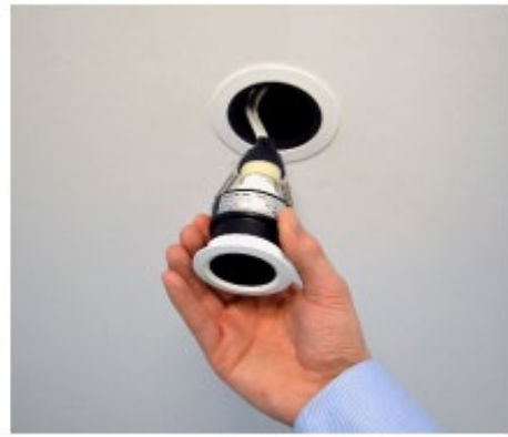
4.4 - Continue until the light hangs freely from its housing
