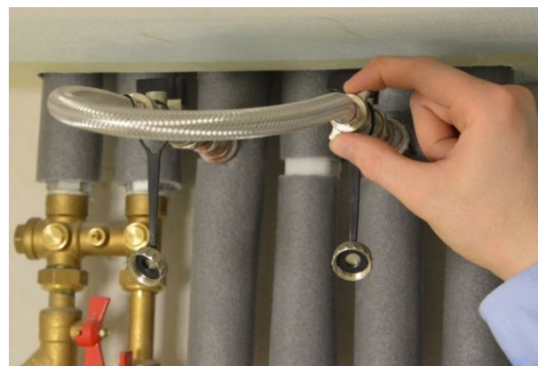
Attaching the loop to the second pipe end
