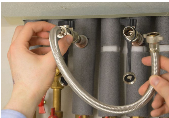
Attaching the loop to the first pipe end
