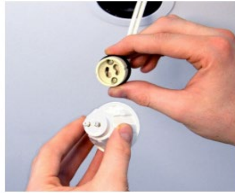
4.8 - release the lamp from the fitting
