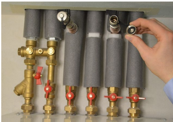
Turn the cap anticlockwise to loosen and remove it
