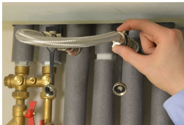
Figure 1.6 Screwing the second end pipe
