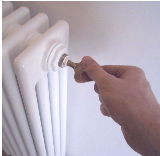
Figure 1.10 Key turning anticlockwise to release the water
