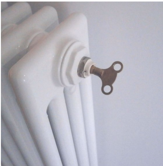
Figure 1.9 Pressure release Radiator key in position
