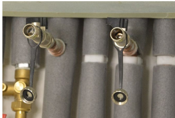
Figure 1.3 Turn the cap anticlockwise to loosen it and remove. Figure 1.4 The pipe caps will get hanging from the valves
