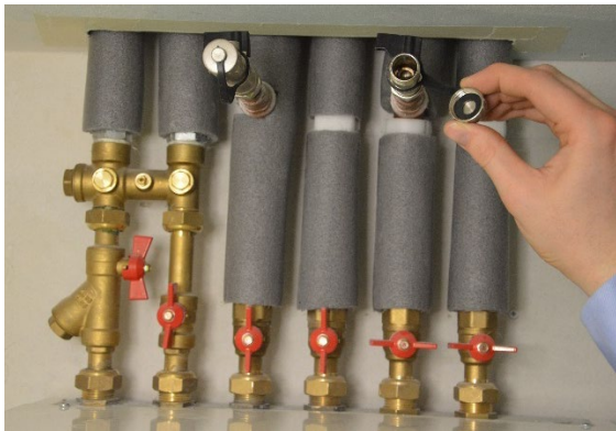
Figure 1.3 Turn the cap anticlockwise to loosen it and remove. Figure 1.4 The pipe caps will get hanging from the valves
