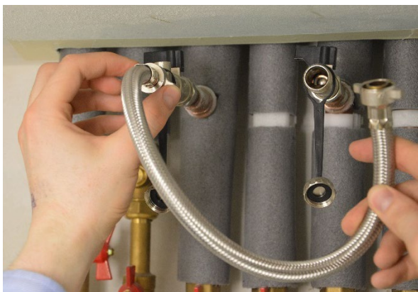
Figure 1.5 Screwing clockwise the first end pipe
