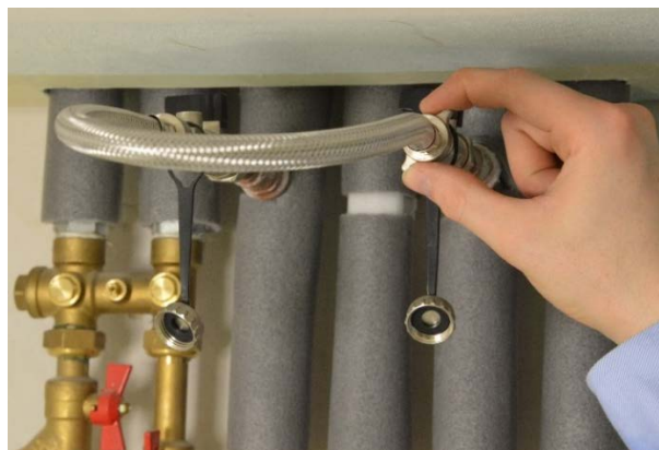
Screwing the second end pipe
