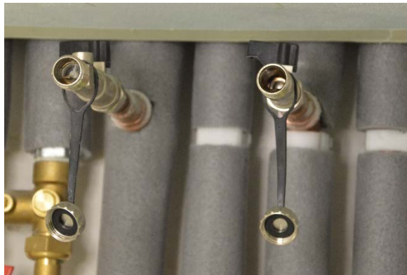
The pipe caps will get hanging from the valves
