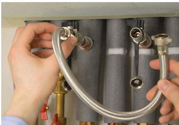
Screwing clockwise the first end pipe
