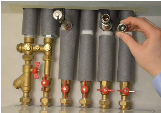
Turn the cap anticlockwise to loosen it and remove.
