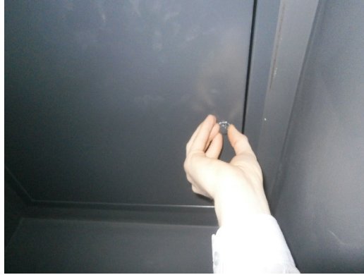
Air Circulating Fan Cupboard Door (Figure 2.2)
