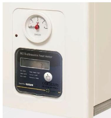
Figure 20 HIU pressure gauge view
